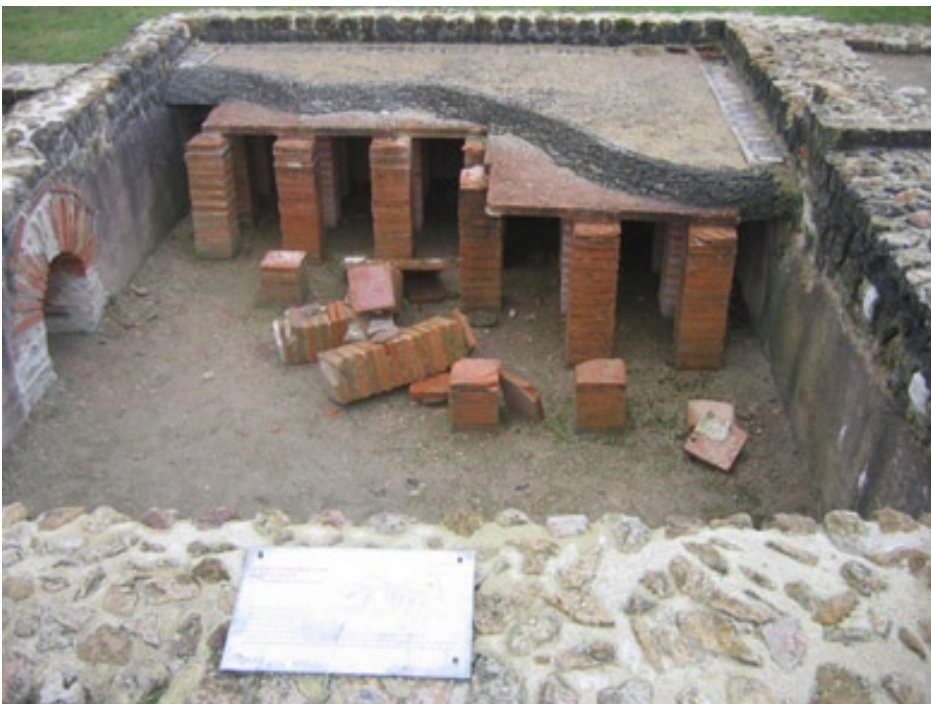
Roman hypocausts used their thermal mass to provide consistent heat to the building above from fires below. source: wikimedia.org
